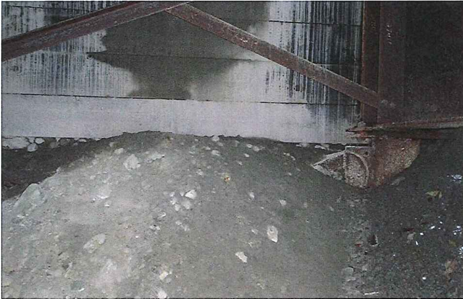
CK2134 Abutment Right Bank
