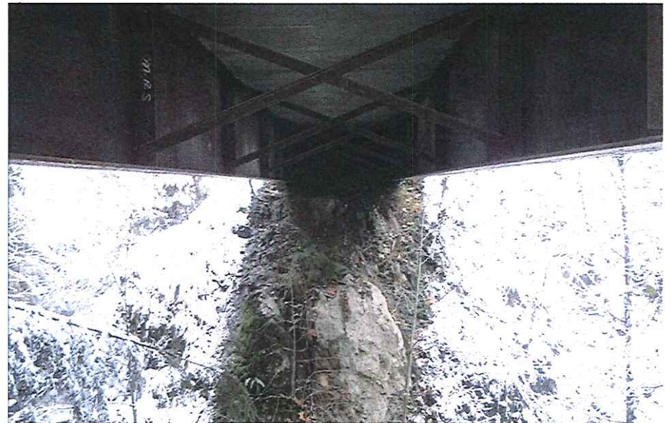
CK2134 Abutment Left Bank
