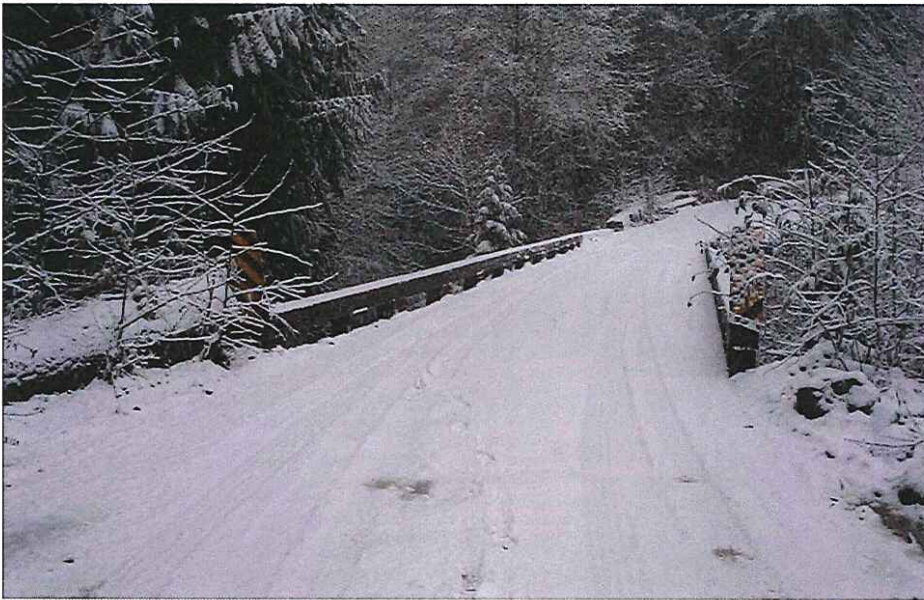
CK2134 Approach Right Bank
