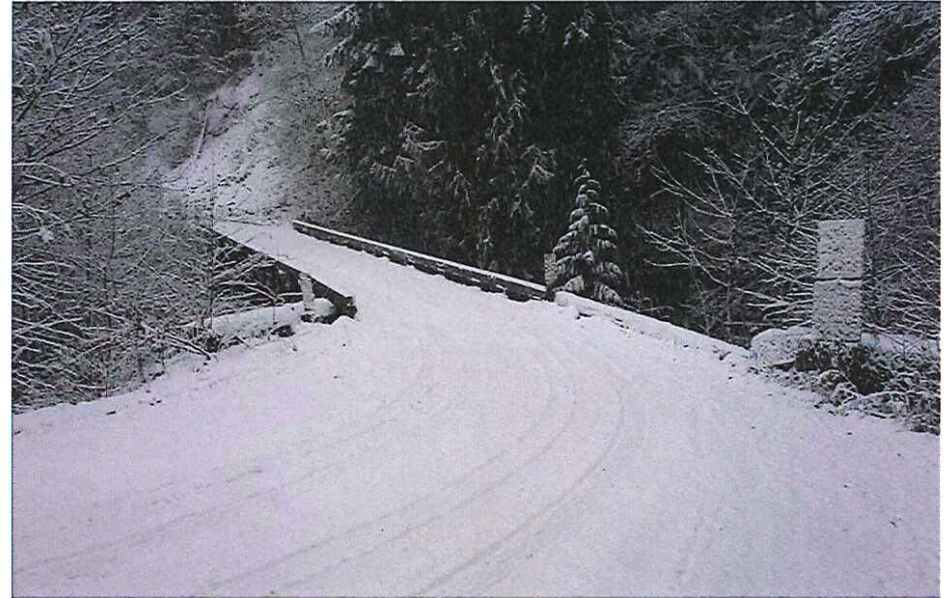
CK2134 Approach Left Bank
